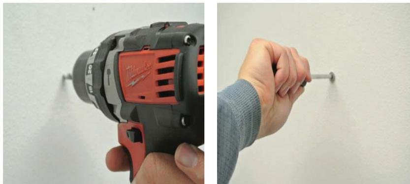
**Figure 3-3 Drilling and Preparing Mounting Holes**
