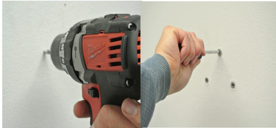
**Figure 7-3 Drill and Prepare Mounting Holes**
