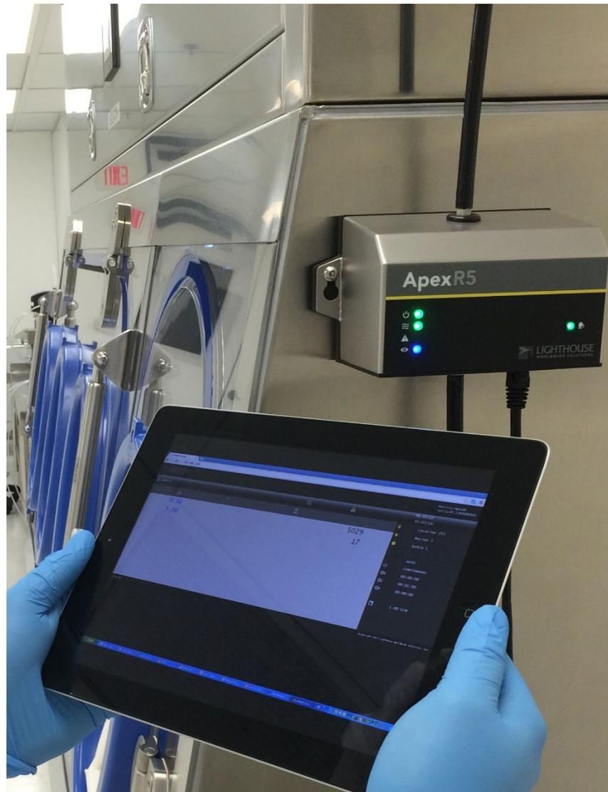
Fig.1 User of EMS system monitoring particle counts in a Cleanroom
