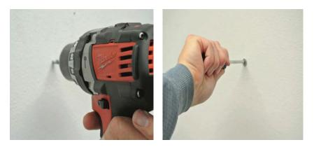
Figure 3-3 Drilling and Preparing Mounting Holes
