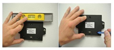
Figure 7-2 Mark Location of Mounting Holes
